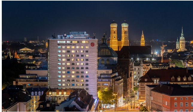
Facade of the NH Collection München Bavaria
