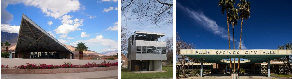
Left to right: Palm Springs Visitor Centre, Aluminaire House (credit Michael Schwarting), City Hall (credit Jake Holt Photography)
